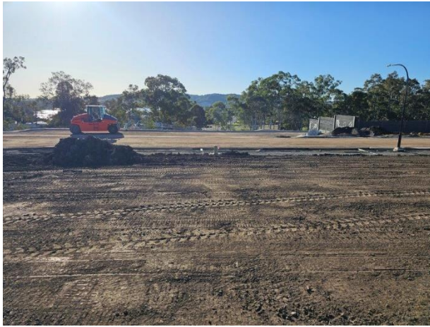
Photograph 3: From Lot 1607, (near BH1601), facing northeast. Showing Outrigger Drive in background.
