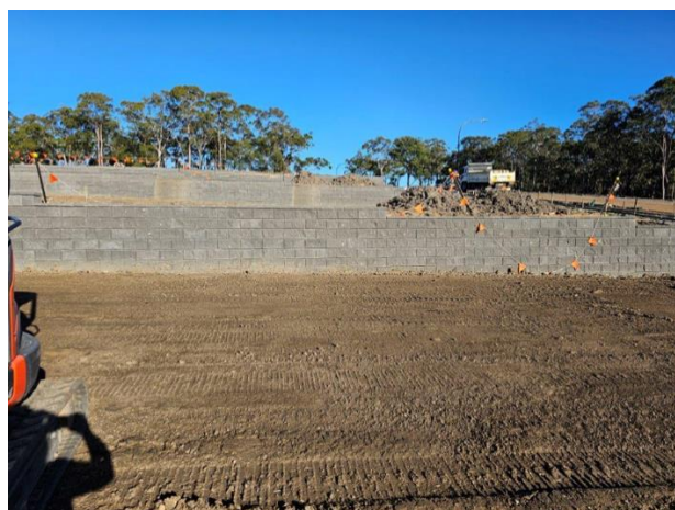
Photograph 1: From Lot 1606, (near BH1601), facing west.
