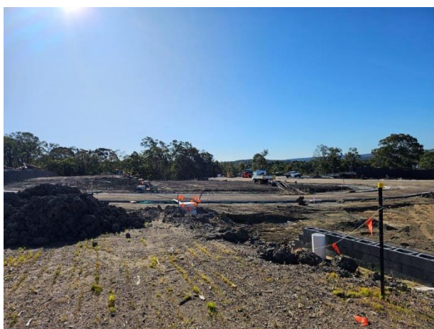
Photograph 11: From Lot 1615, (near BH1609), facing north.
