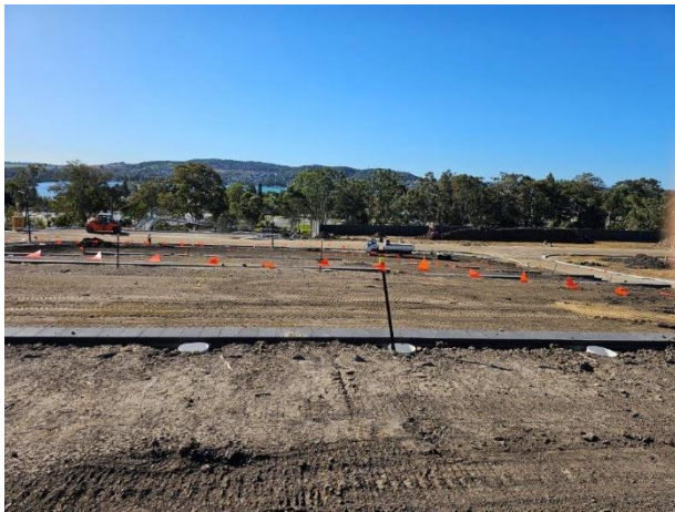
Photograph 5: From Lot 1612, (near BH1606), facing east.
