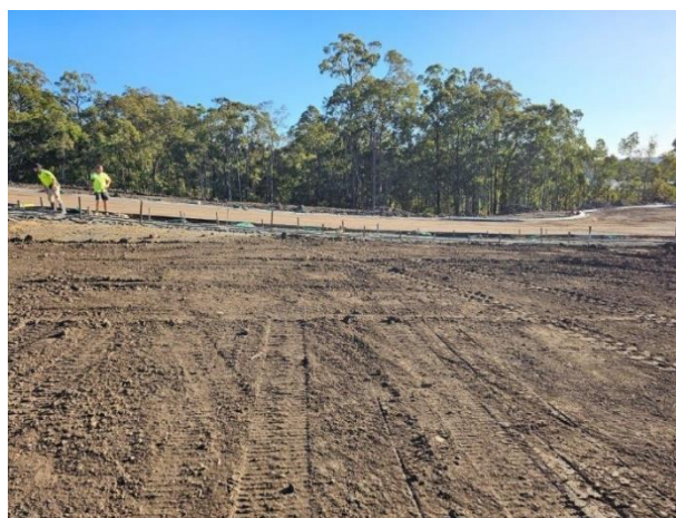
Photograph 2: From Lot 1606, (near BH1601), facing north.
