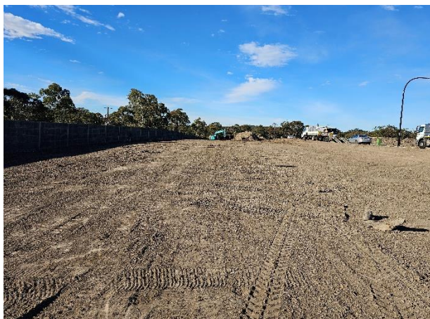
Photograph 1: From boundary of Lots 2401 and 2402, (near BH2401), facing south.
