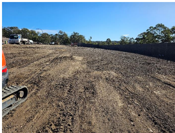
Photograph 4: From boundary of Lots 2407 and 2408, (near BH2404), facing northwest.
