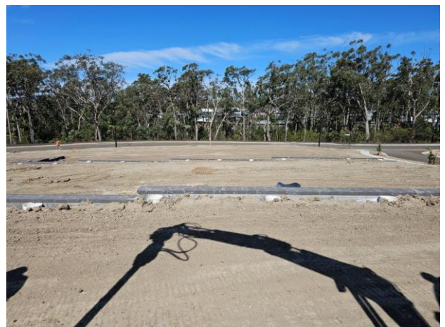
Photograph 6: From near BH1012 (Lot 1012), facing south.
