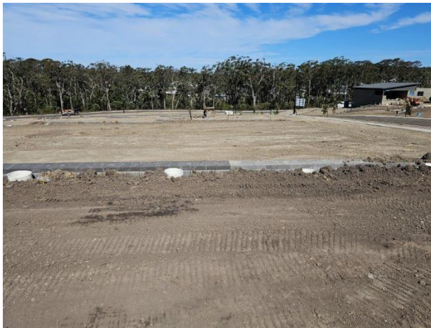
Photograph 3: From near BH1008 (Lot 1008), facing south.
