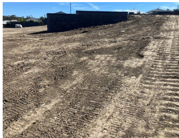
Photograph 8: From near BH1903 (Lot 1904), facing west.
