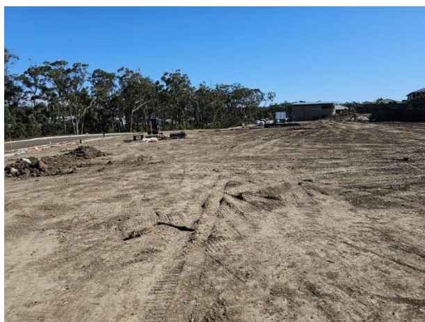
Photograph 9: From near BH1905 (Lot 1902 / 1903 boundary), facing west.
