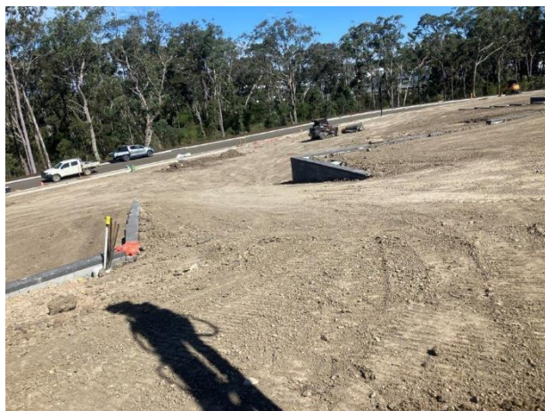
Photograph 7: From near BH1903 (Lot 1904), facing southwest.
