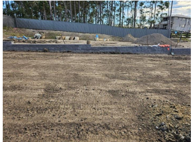
Photograph 2: From near BH1002 (Lot 1007), facing north.
