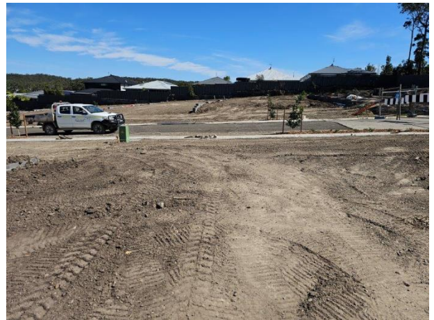
Photograph 4: From near BH1008 (Lot 1008), facing west.
