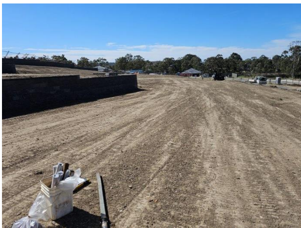
Photograph 5: From near BH1012 (Lot 1012), facing northeast.
