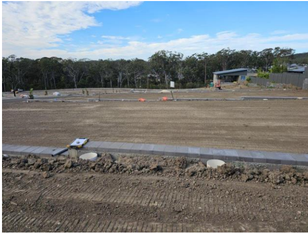
Photograph 1: From near BH1002 (Lot 1007), facing south.
