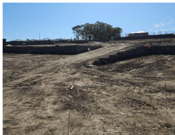
Photograph 10: From near BH1905 (Lot 1902 / 1903 boundary), facing northwest.
